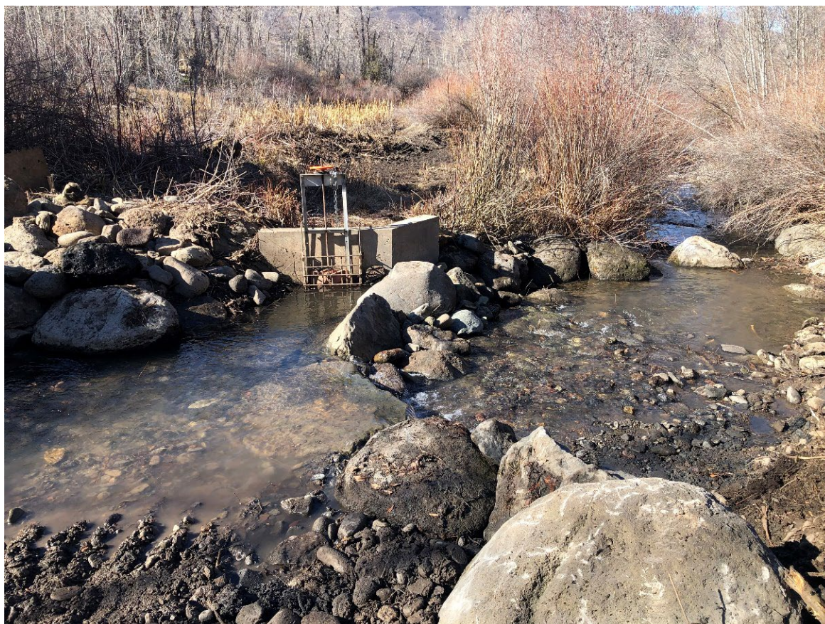
Photograph 8. Reconstructed diversion system, Fourmile Creek, November 13, 2023.
