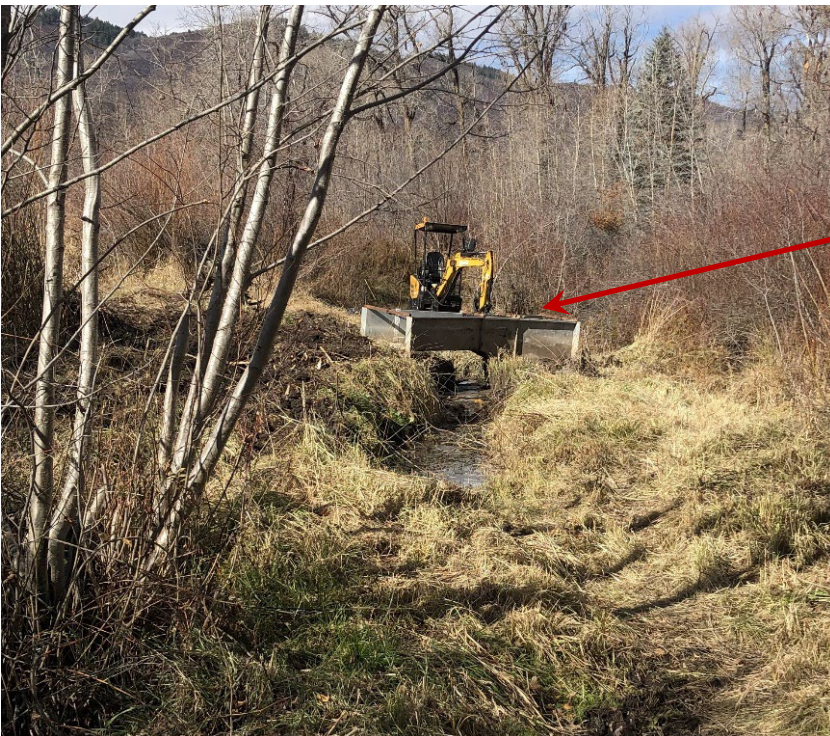
Photograph 2. Parshall flume is removed from ditch.
